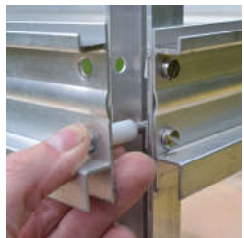
Nylon spacer on bolt
