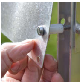
Plastic spacer on infill plate
