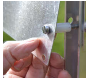
White spacers on infill plate
