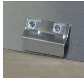
Completed bracket inside the frame
